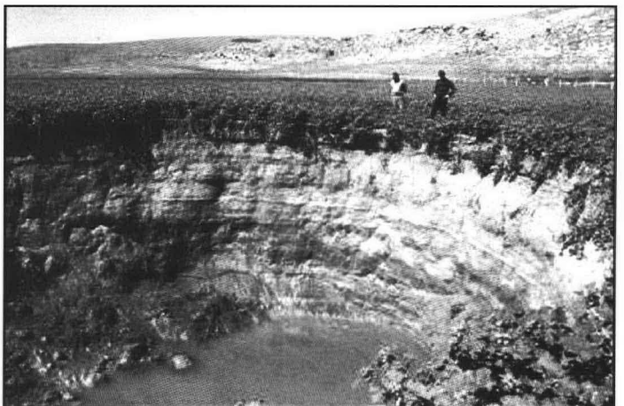
Figure 8 The second sinkhole viewed of from the southwest. The reservoir area outside the minimum capacity area is covered by natural vegetation due to the fact that it contains no water. The photograph was taken in October 2002, 7 months after the formation of the sinkhole.
